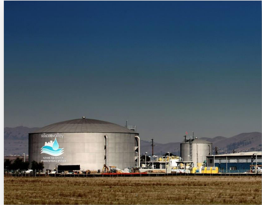
Silicon Valley Advanced Water Purification Center
