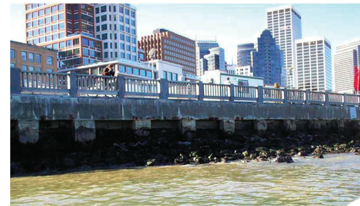
Seawalls (Grey Infrastructure)
