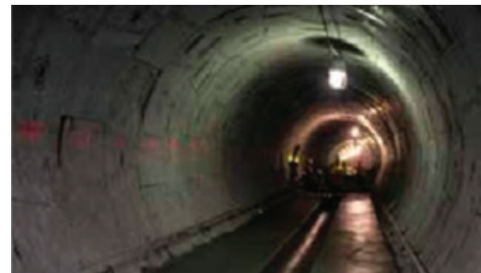
Storage Tunnels (Grey Infrastructure)
