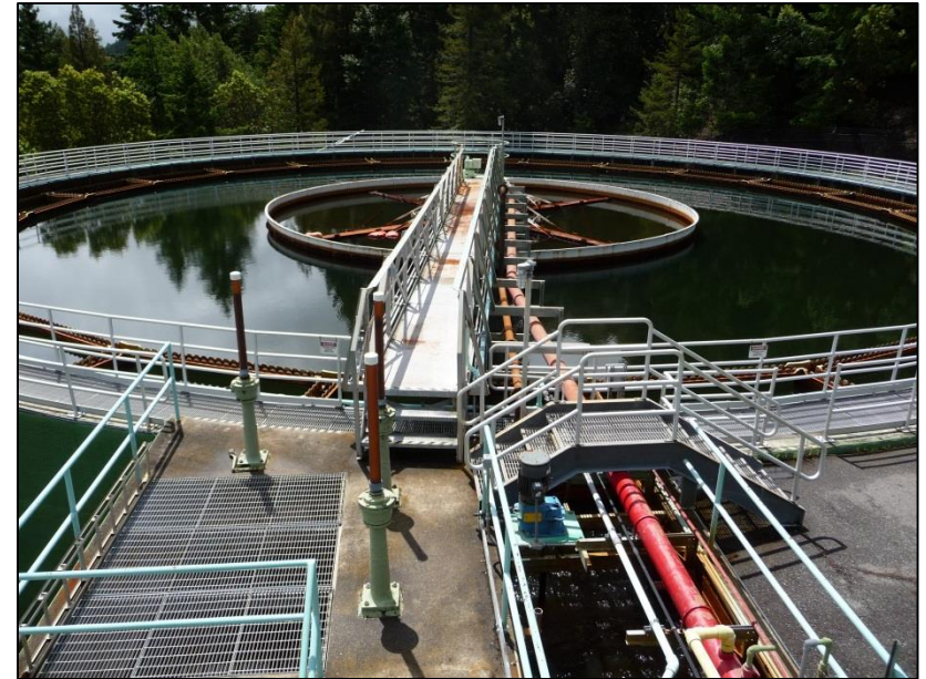
Bon Tempe Treatment Plant
