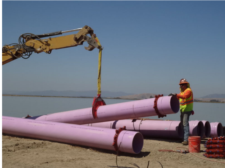
Purple pipe being installed for the North Bay Water Reuse Program. (Photo Credit: North Bay Water Reuse Authority)
