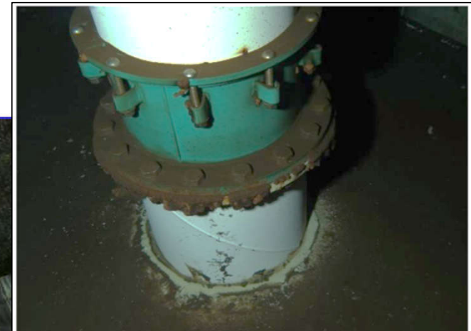
Minor galvanic corrosion on inlet pipe flange (interior of tank)
