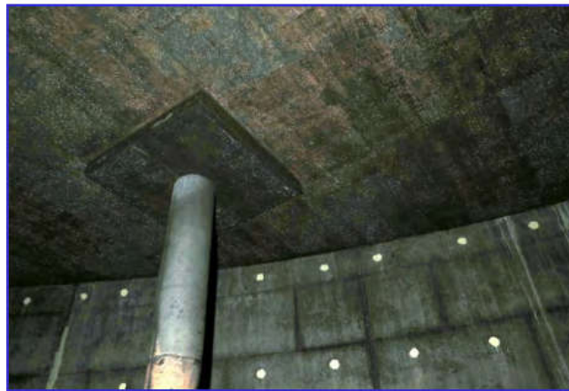
Concrete support column (interior of tank)
