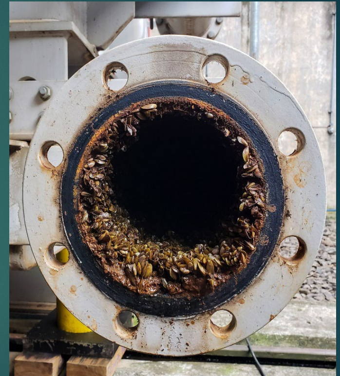
Golden mussels colonizing a water pipe at a hydroelectric plant in Brazil (Mountinho, 2021).
